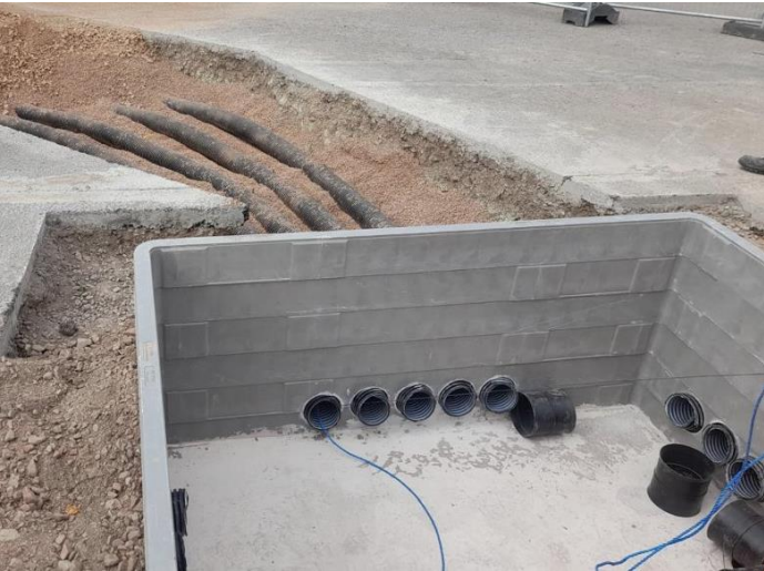
Figure 15 – Equipment base and provision for cabling under construction on a depot site
