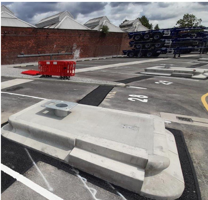
Figure 5 - Charging bays under construction for Maritime
