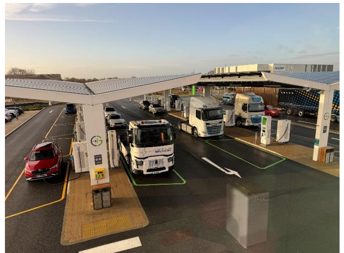
Figure 4 - eHGV tractors at GRIDSERVE Electric Forecourt®, Braintree
